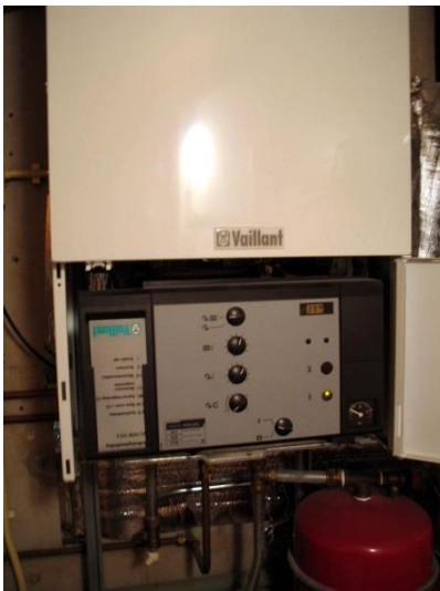
Closed type CV boiler. Source figure: Dutch wikipedia CV boiler site.
